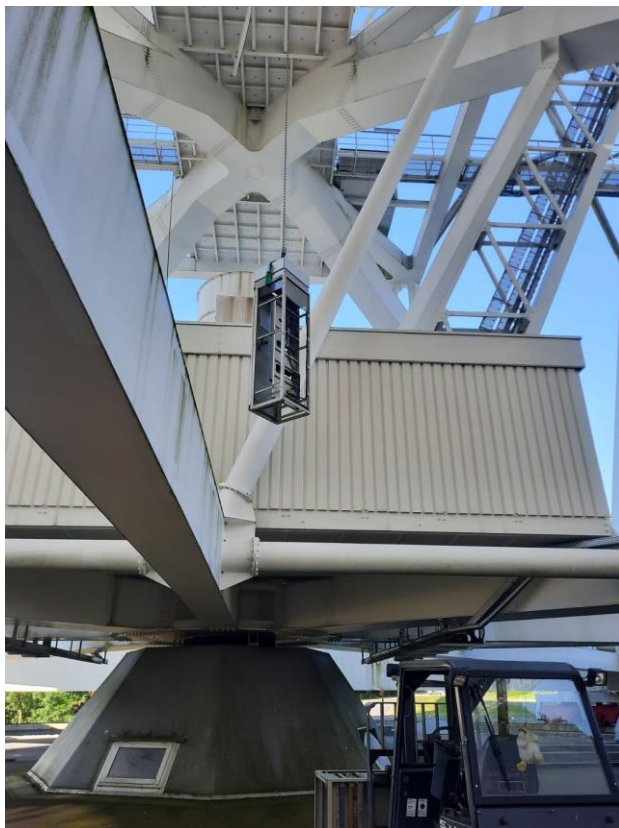
Installation of the new racks in the telescope (picture by H. Homburg).
