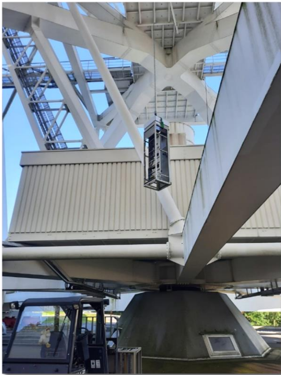
Installing new racks for the drive control in the telescope (Andre Bauerfeind, MPIfR)
