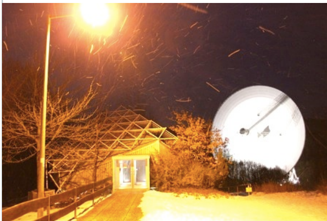
The visitors' pavilion in a winter environment. In the neighbourhood of the pavilion we have three astronomical walks at different scale (Planetary Walk, Milky Way and Galaxy Walk). The access to the viewing spot in direct vicinity of the 100m radio telescope is rebuilt at the moment to become accessible also for people with impairments.
