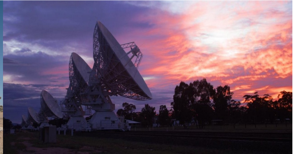
ATCA, Paul Wild Observatory, Australia Six 22-m telescopes, 86 GHz Calibrator sources 1253-055, 1921-293 and Uranus
